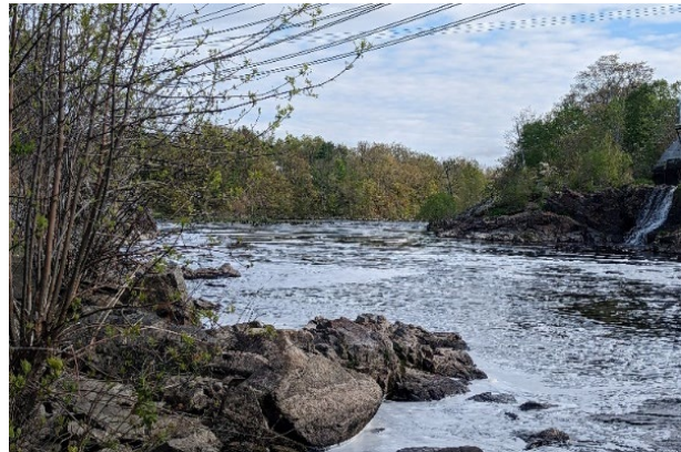
Figure 1: Tailrace of the Milltown dam looking downstream from the fishway entrance.
