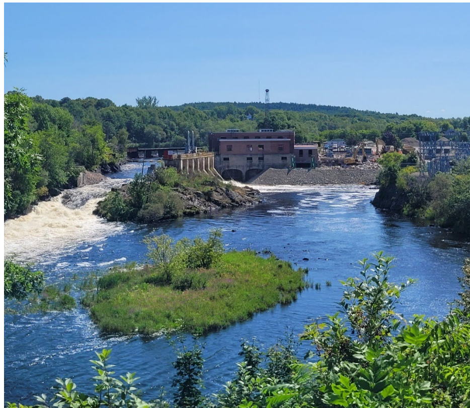
Figure 9: Milltown Generating Station (MGS) decommissioning as of August 23, 2023
